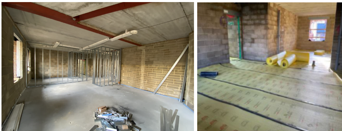
Internal fit out underway on plots 53/54 (Feb 2023)
