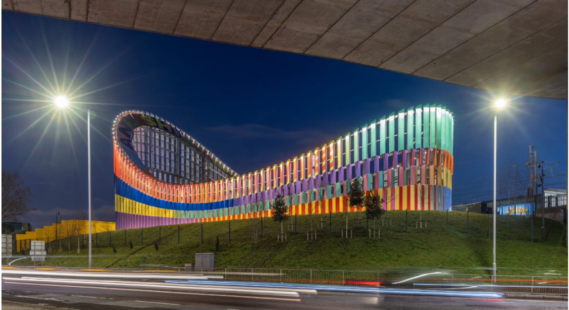
Brent Cross Town primary substation
